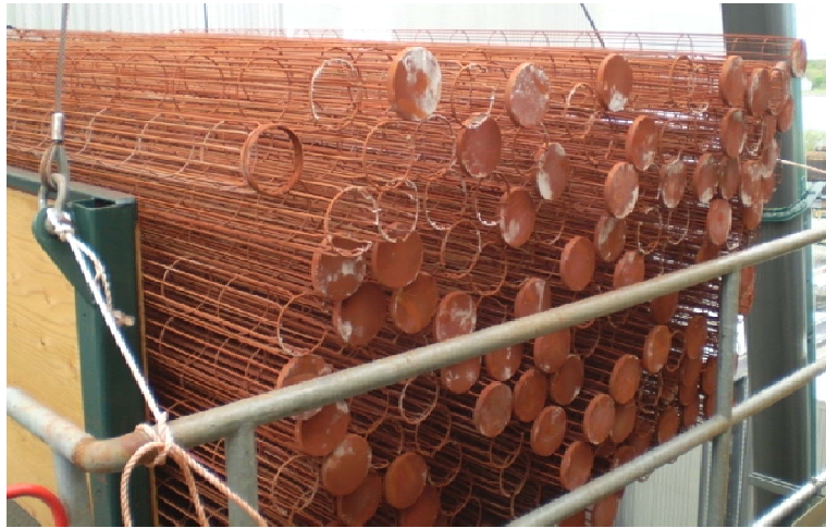
Replacement of PJFF Old Cages
