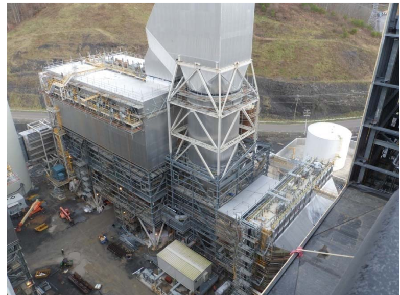
PJFF Installation with CDS
