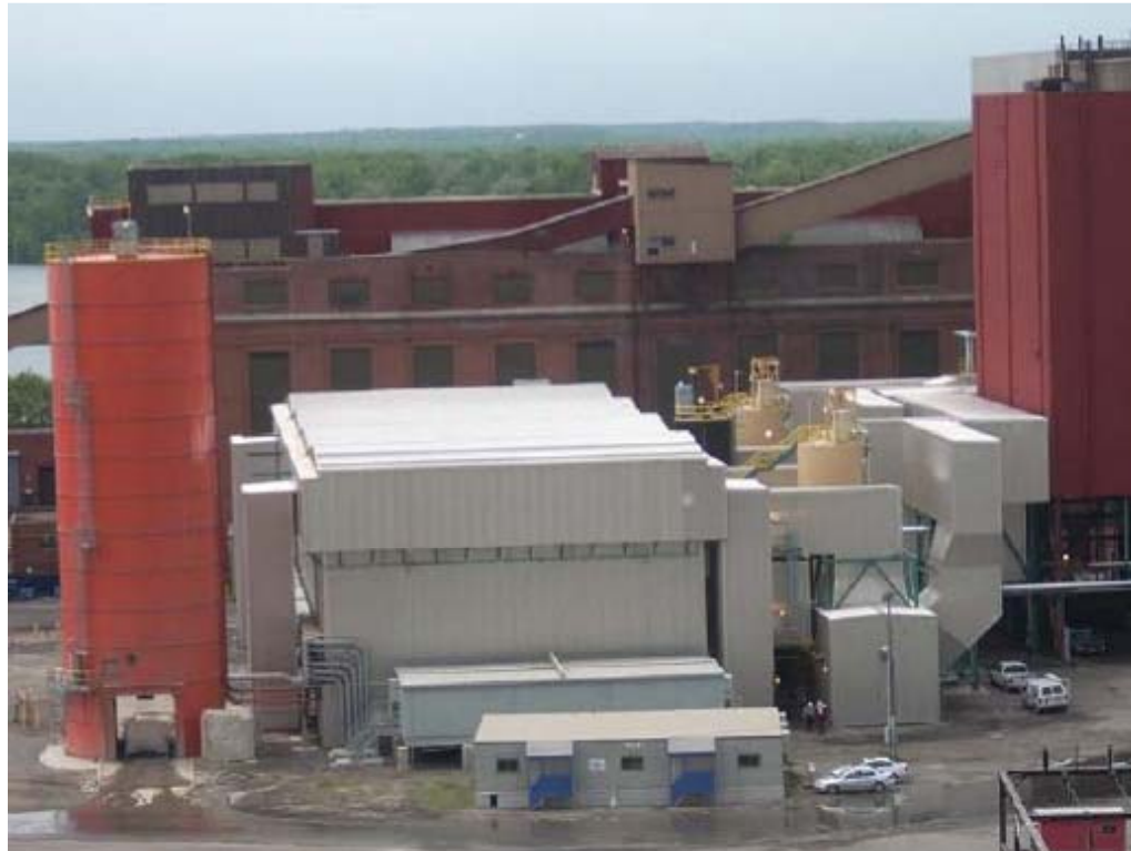
Trona Injection DSI FGD-PJFF
